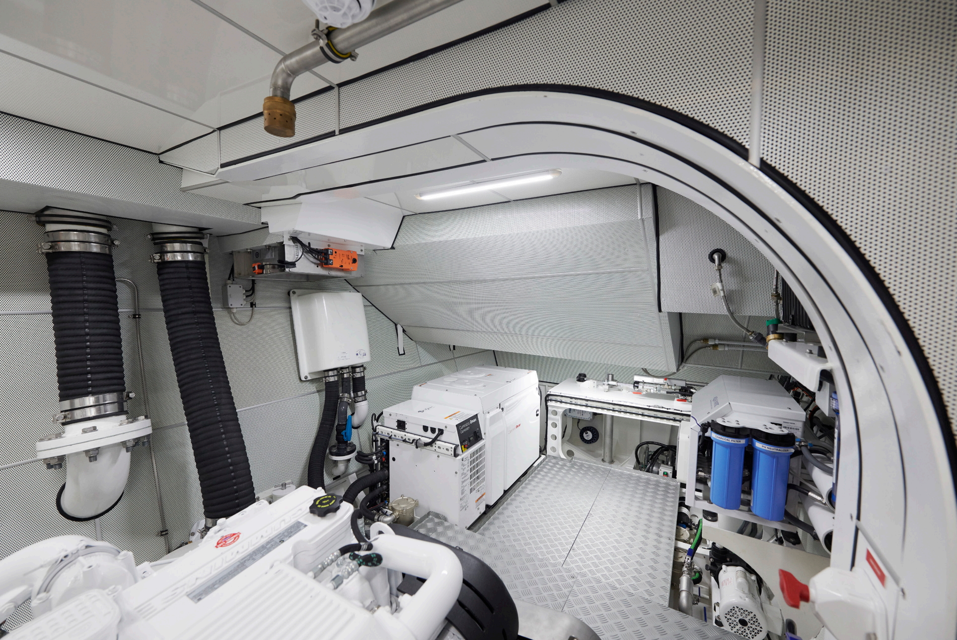
Starboard engine room
